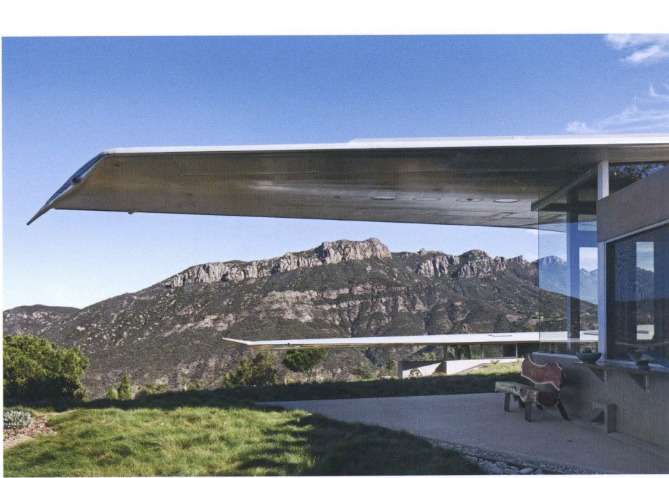
End of wing 翼の端部
