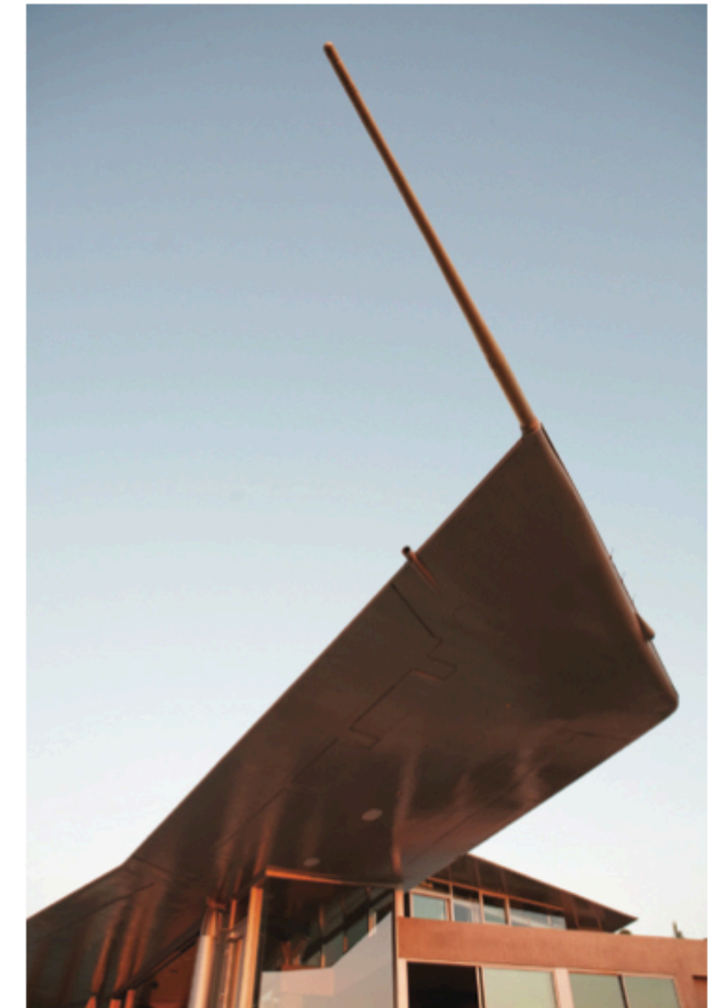
ABOVE AND ABOVE LEFT: The Wing House in Malibu, so-named for its roof, which Hertz constructed from the wings of a decommissioned Boeing 747.
