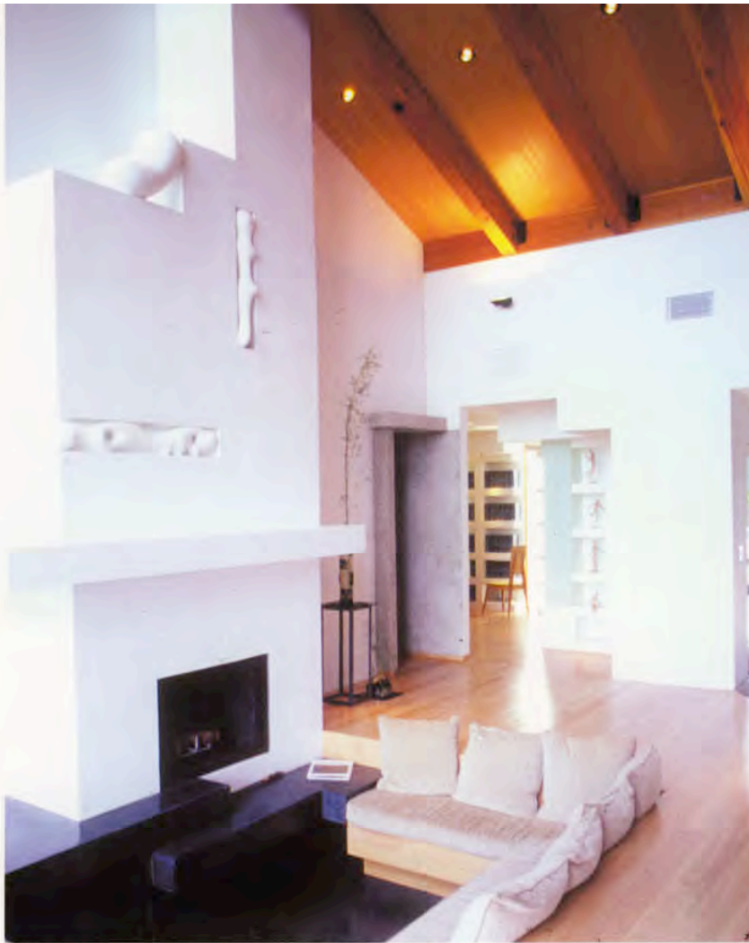
The roof of the living room and master bedroom (left) are constructed out of recycled timbers, detailed to create an exposed and honest expression of the framing and structural system and their connections.
