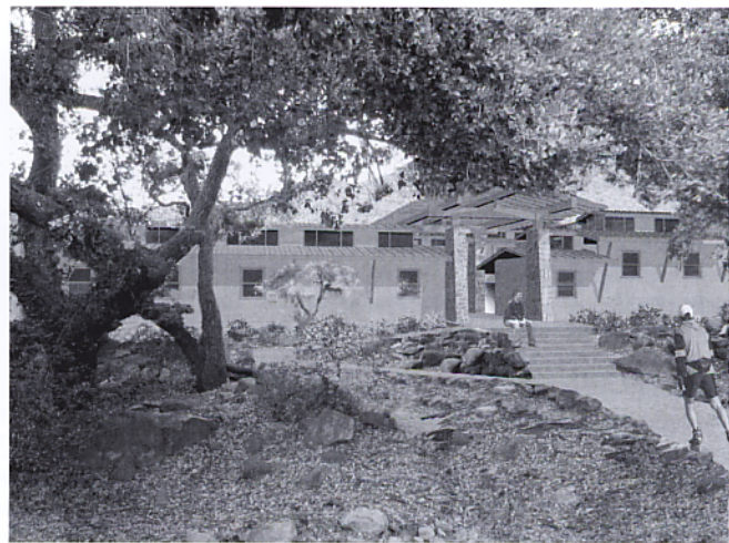
Main approach to Lower School from the south
